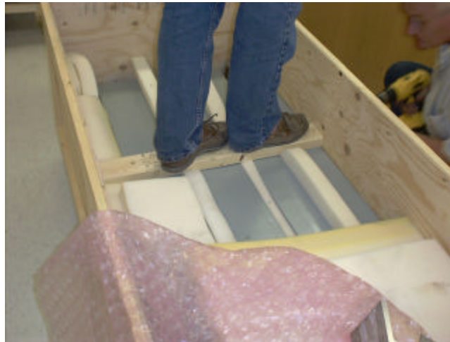
Fig. 3: 2"x4" sections preventing up-down motion of I-beams
