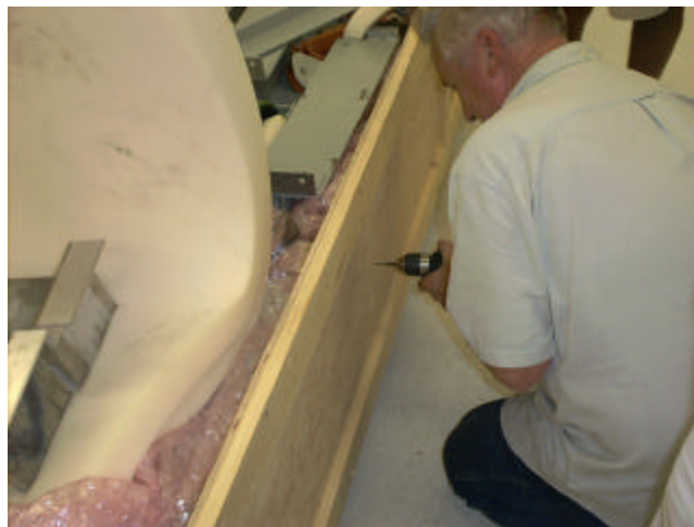
Fig. 4: 3/8" plywood sides with 1"x4" frame members
